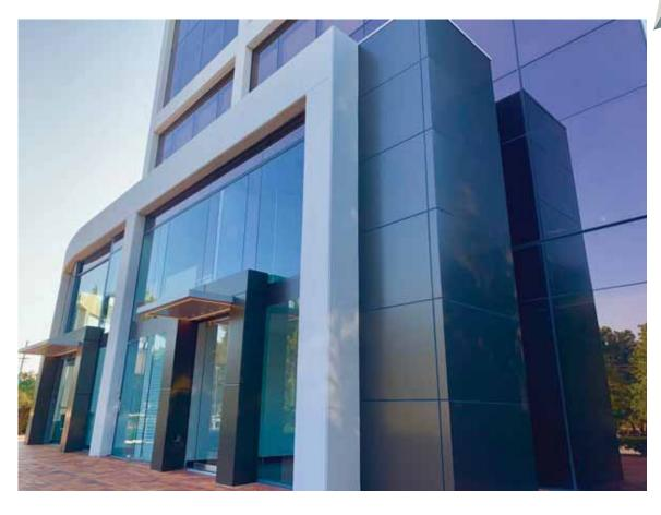
ACP-FR Aluminium panels have good performance such as light weight, high strength, stiffness, structural stability, manufactured from high grade aluminium, with a surface finish which uses the advanced technique of fluorocarbon lacquer pre-coil coating.
